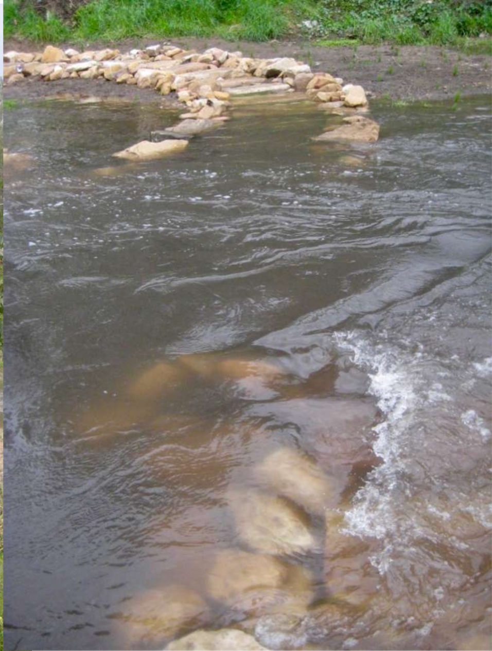
New stepping stone crossing, Toongabbie Creek – impassable with even minor flooding
